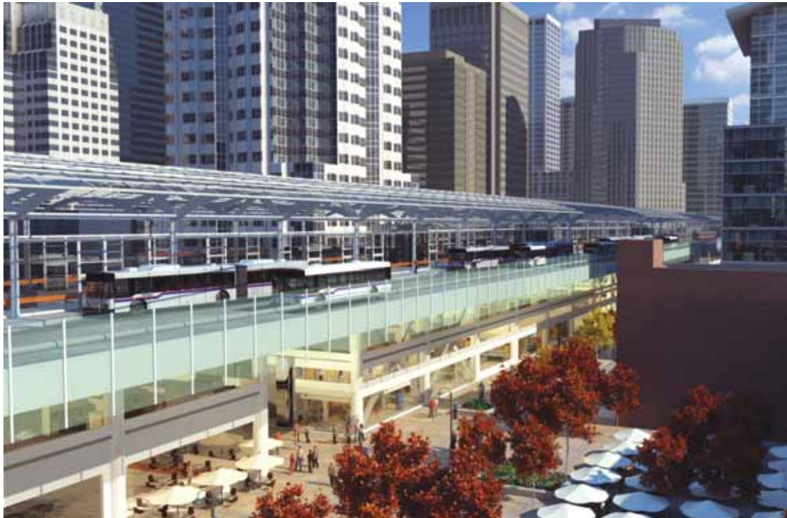
Opposite: Image of high speed rail running along Union Pacific Rail Road lines through Central California. Above: San Francisco's TransBay Terminal. Both images courtesy NC3D. More images of the California High Speed Rail project are available at http://www.nc3d.com/projects/california-high-speed-rail-2.html .
