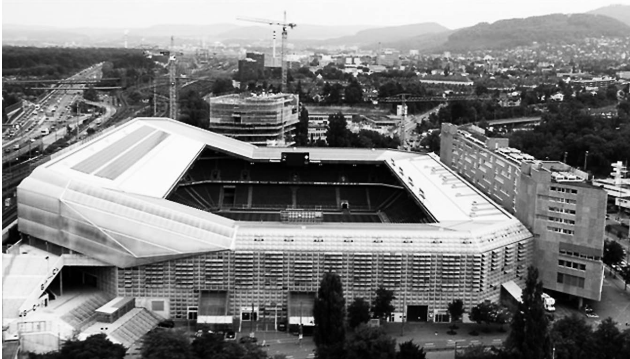
Mixed Use Project: Senior Living, Sports Arena, and Shops, St. Jacob's Park, Basel, Switzerland, Architects: Herzog and deMeuron. Photo ©Euro 2008 SA.
